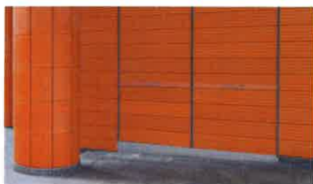
Contemporary interpretation of heritage brick buildings - terracotta scaled brick rainscreen
